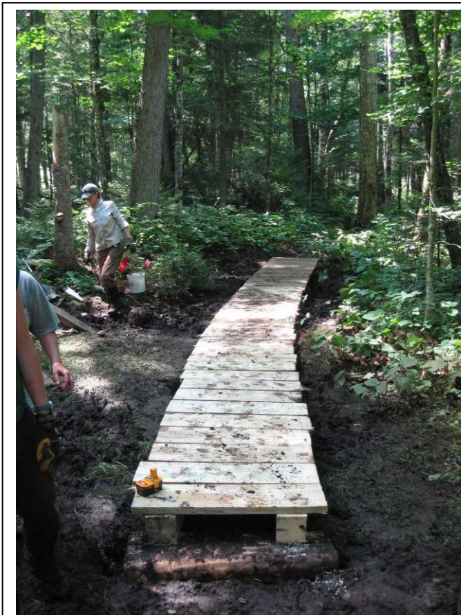
Bog bridging constructed by the NFCT Stewardship Crew in 2010.
