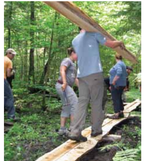
Laying bog bridging; Attean Pond, ME.
